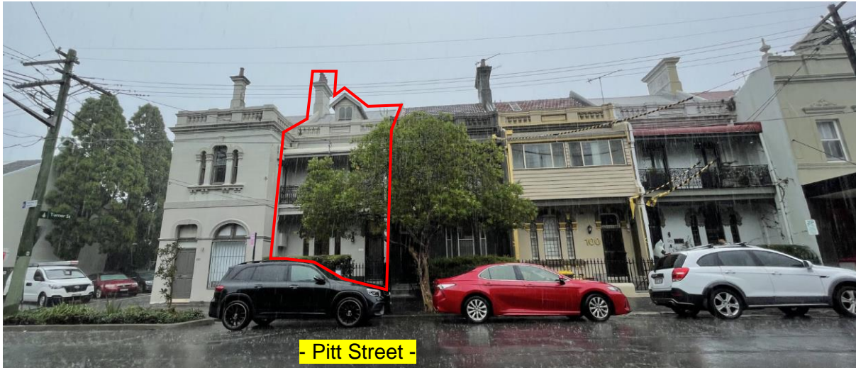
Figure 4: Site viewed from Pitt Street (source: Council Planning Officer - 20 February 2024)
